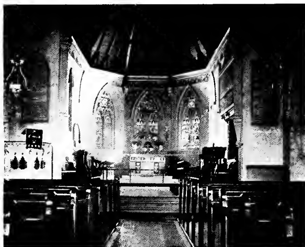
VIEW SHOWING DEFECT IN ORDINARY APSE. THE CENTRAL WINDOW LOOKS LOWER THAN THOSE ON EITHER SIDE
